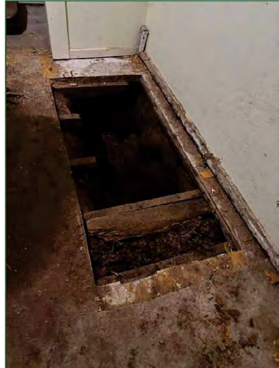
Photo 7 – Compromised Wood Floor with Open Sanitary Drain
