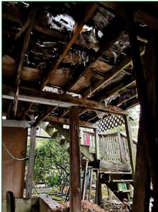
Photo 22 – Compromised/Rotted Deck Joists and Plank at Rear Entry
