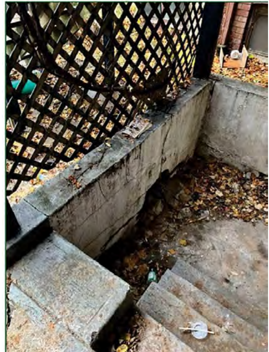
Photo 4 – Collapsed Walkout Wall
