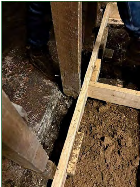
Photo 14 – Rotted Stud at Base of Load Bearing Wall
