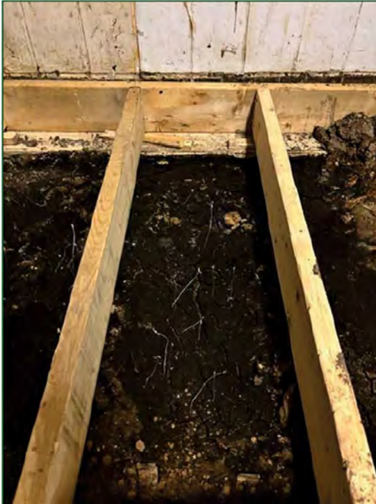
Photo 17 – Vegetation Growth at Floor Infill
