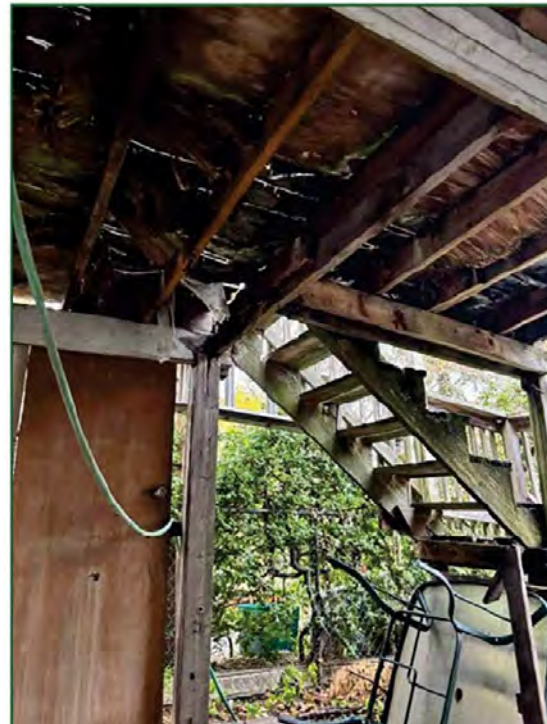
Photo 24 – Compromised/Rotted Deck Joists and Plank at Rear Entry
