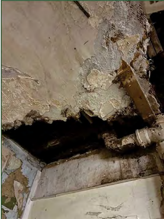
Photo 13 – Moisture Damaged Floor Joists
