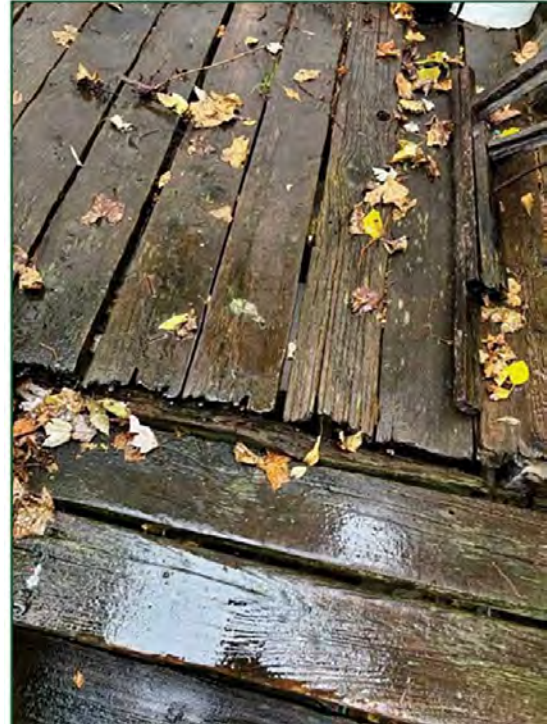
Photo 31 – Rotted Deck Boards at Rear Stair
