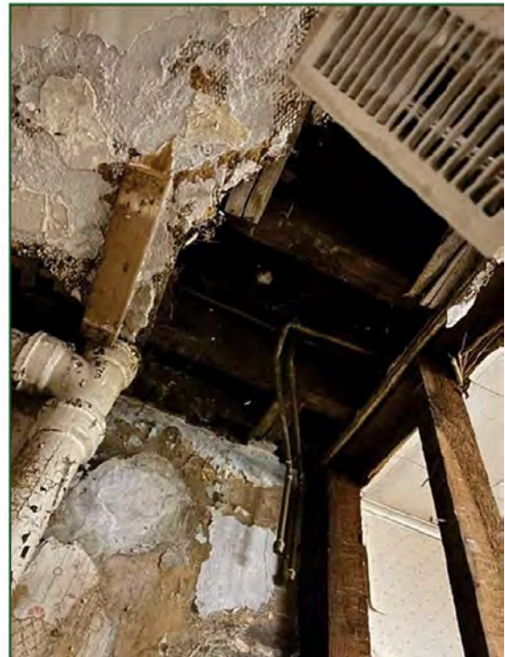
Photo 12 – Moisture Damaged Floor Joists
