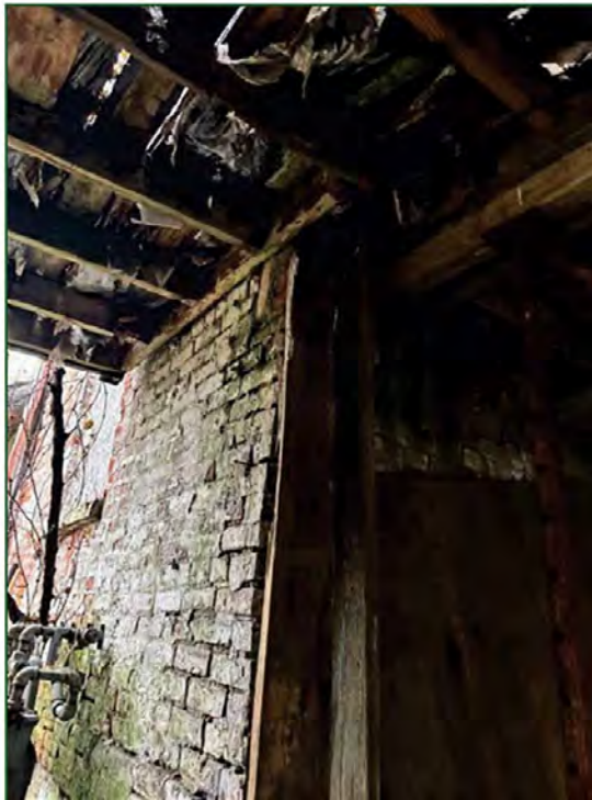
Photo 25 – Cracked/Settling Brick Wall at Rear Addition
