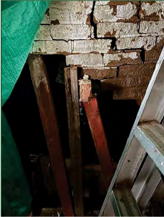
Photo 37 – Poorly Shored/Failing Opening in Brick Wall at Rear Addition
