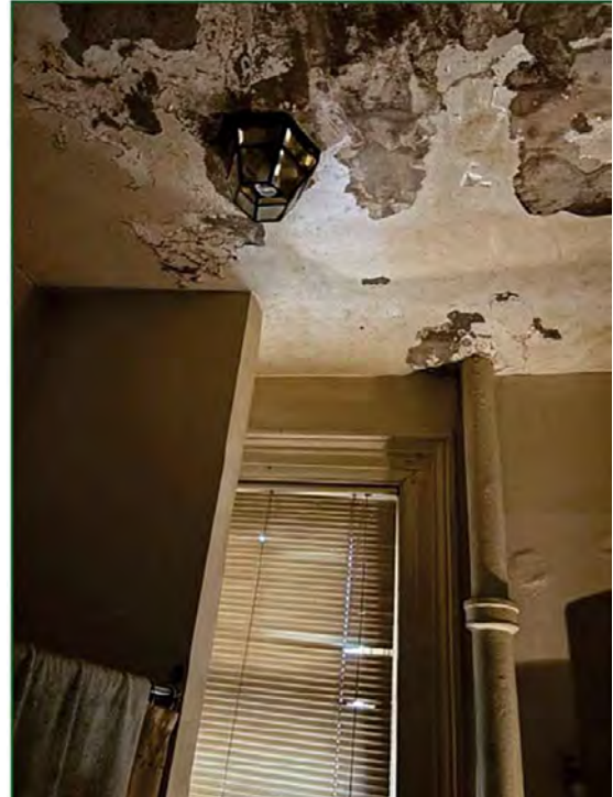
Photo 39 – Moisture Damage in Ceiling
