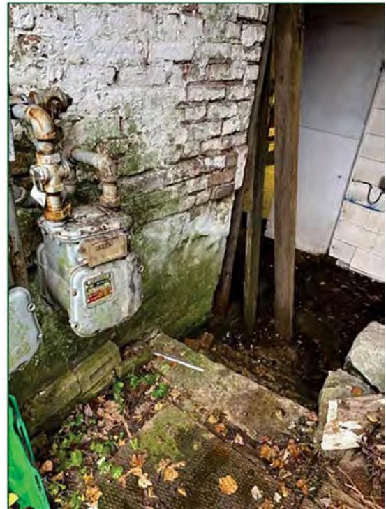
Photo 27 – Cracked/Settling Brick Wall at Rear Addition
