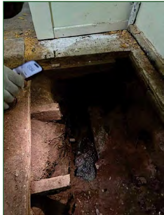
Photo 8 – Compromised Wood Floor with Open Sanitary Drain
