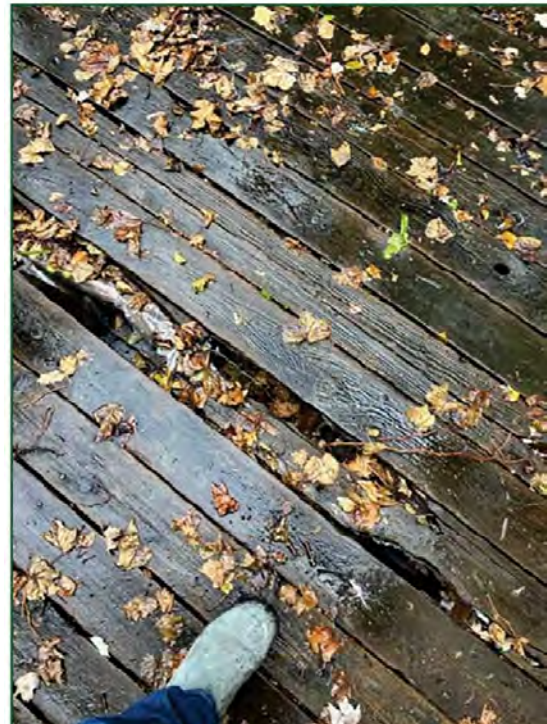
Photo 32 – Rotted Deck at Rear Stair
