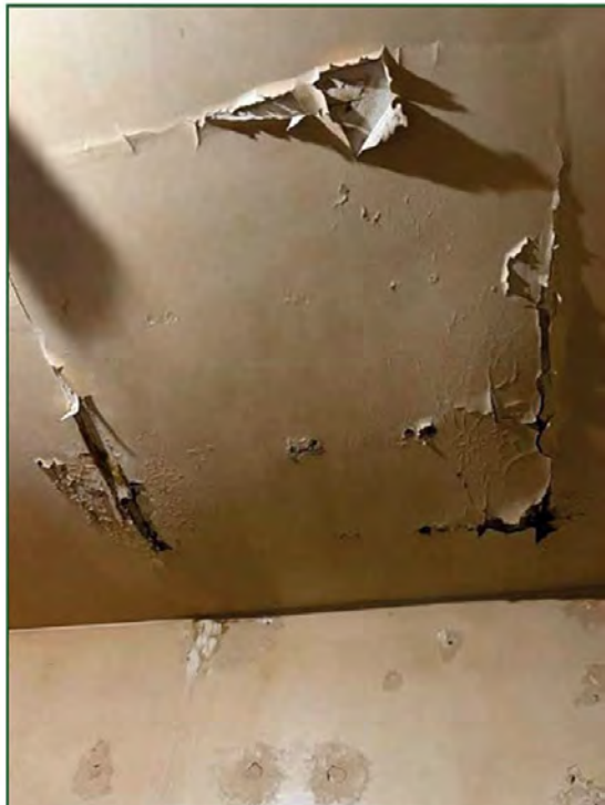
Photo 38 – Moisture Damage in Ceiling
