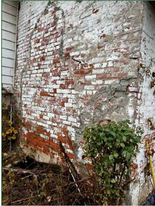
Photo 29 – Cracked/Settling Brick Wall at Rear Addition
