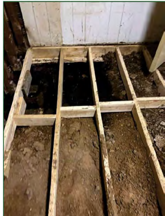
Photo 16 – Re-Framed Wood Floor on Soils with no Isolation
