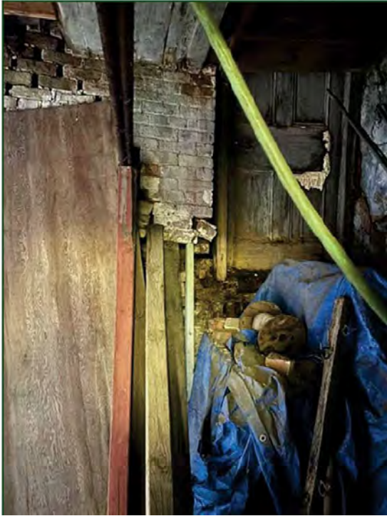
Photo 21 – Collapsing Brick Wall at Rear Entry
